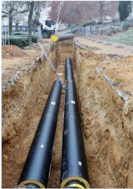
Execution of the works on the Valladolid heating network
