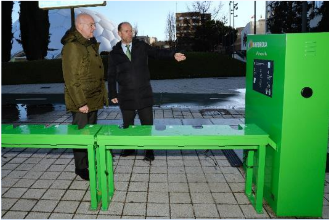
Electric vehicle charging stations in the Millennium Dome area.
