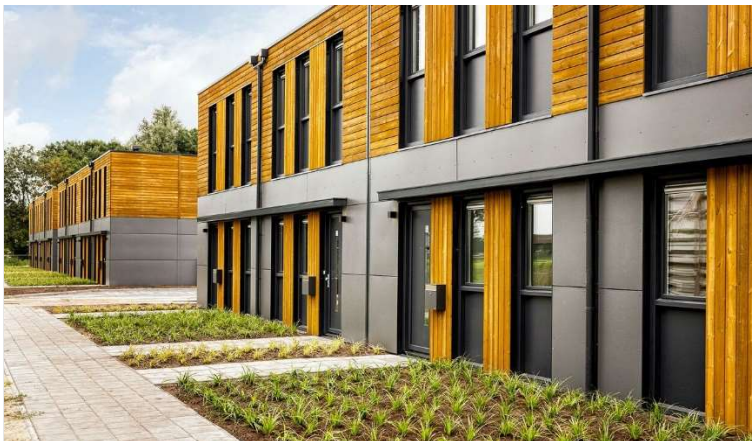
Figure 15 Temporary homes in the village of Ten Post
