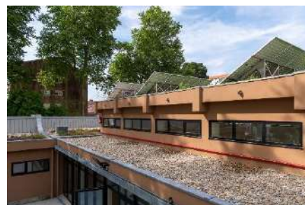
Figure 41. Renovated Falcão school.
