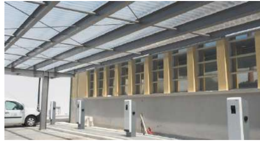
Figure 37. Águas e Energia's charging park.
