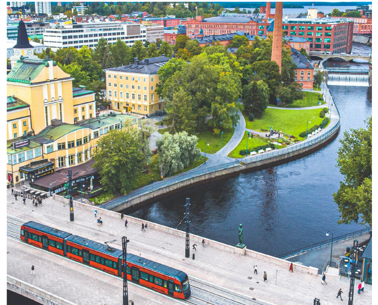
Image 2. It should be borne in mind that many measures set out in the roadmap are also often taken for reasons that are not purely climate-related. The other benefits include a more comfortable, healthier and safer environment, the commercial opportunities brought about by technologies, the economic sustainability made possible by life-cycle thinking, and increased biodiversity. Image: Laura Vanzo.
