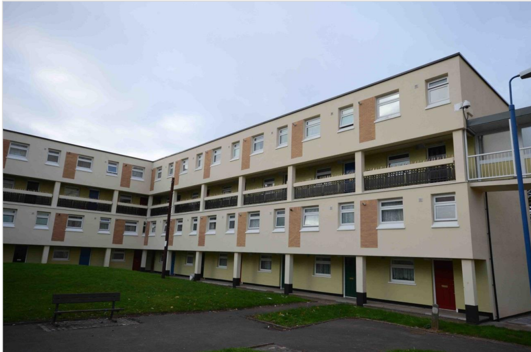
Example of ELENA-BRITE actions: a tower block building after refurbishment (Picture courtesy of the Bristol City Council)
