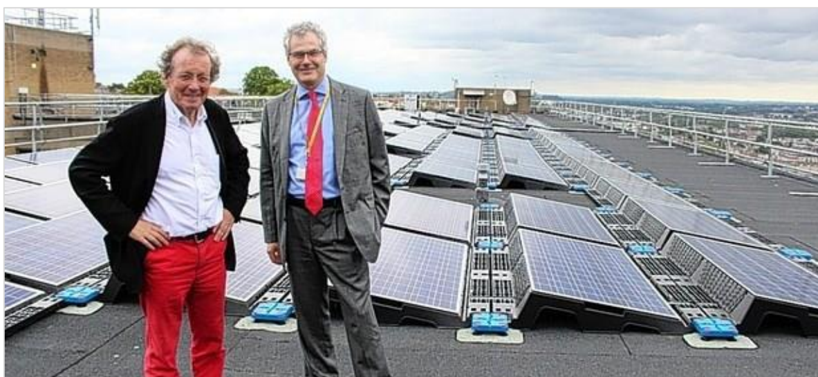
Example of ELENA-BRITE action: installation of rooftop solar PV on St. Michael's hospital - 50kW (Picture courtesy of the Bristol City Council)
